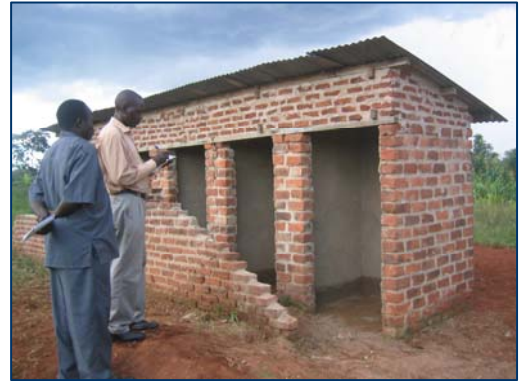
Pit latrines constructed by parents of Wangobo P/S, Bugiri District
