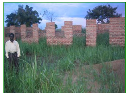
Teachers houses under construction Mutere P/S Mayuge District
